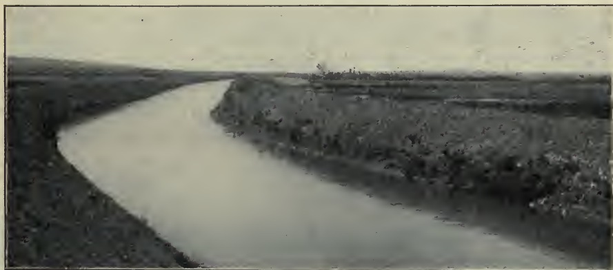
FIG. 47. — A large ditch, in western United States, in which water is led from a river to be used in watering crops by irrigation.
